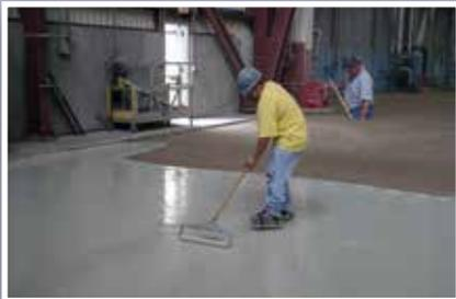
Penntrowel® Systems trowellable, slurry-broadcast, and laminate polymer linings provide durable corrosion protection for floors and other concrete structures.
